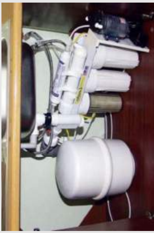
Filters fixed under the sink
